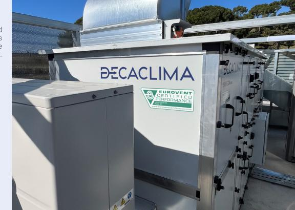
Outdoor unit and AHU connected as standard to save pipe work.
