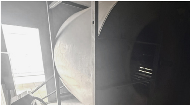
Initial client installation
